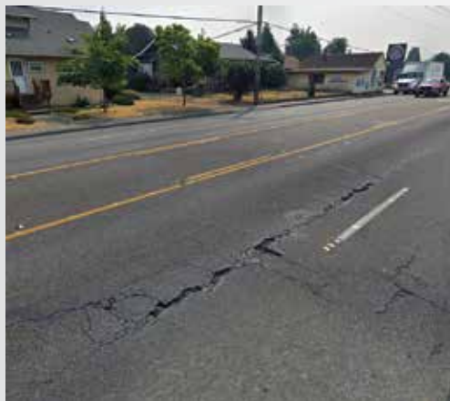
Existing Condition: A St. SE near 7th St. SE
