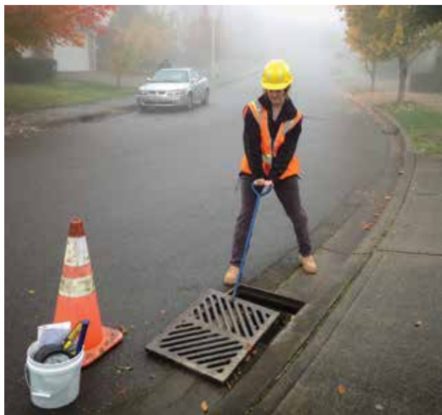
A storm catch basin being inspected by City of Auburn storm technicians. You will see them in the street, near the sidewalk in front of your home or business. They usually have a grate covering them.
