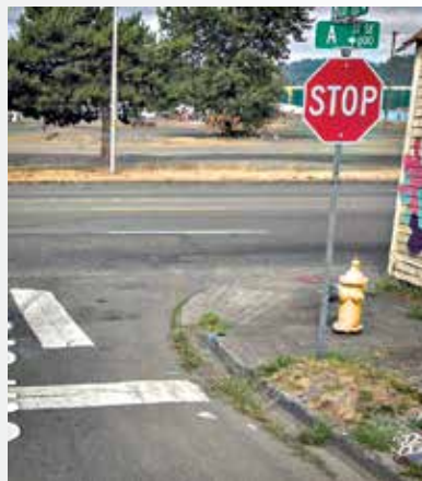
Existing Condition: A St. SE & 8th St. SE
